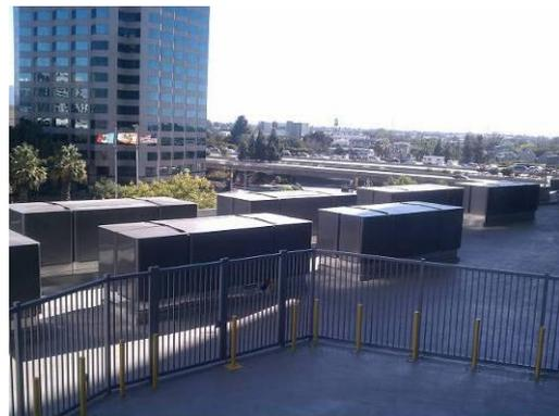
Adobe gave a very interesting paper on how a building energy management system significantly cuts electricity demand and costs at its headquarters in San Jose, California. The key is to synchronise the switching of the various loads to minimise overlap and reduce peak demand. Bloom Energy's 1.2 MW fuel cells provide approximately a third of the electricity requirements at Adobe's HQ.
